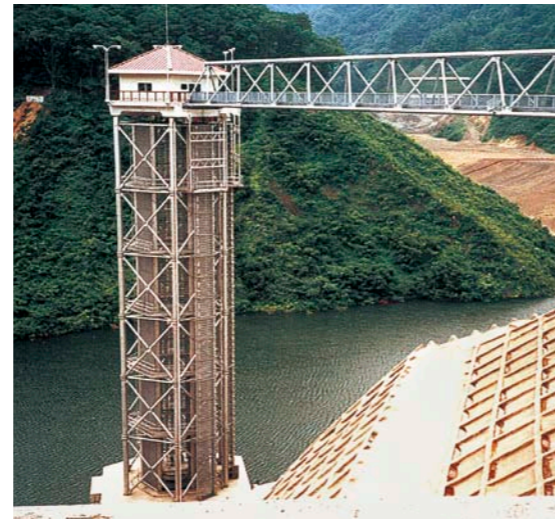
Dam's head gate tower (304)
