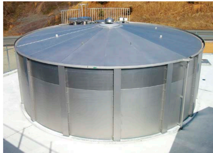
Water supply plant (304, 316, SUS329J4L)
