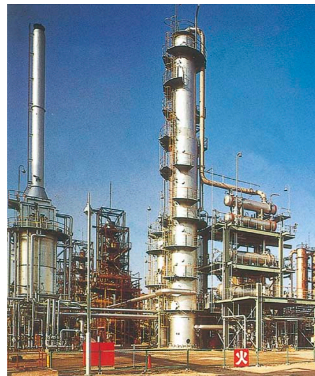
Petrochemical plant (304, 316L, S31803, e.t.c.)
