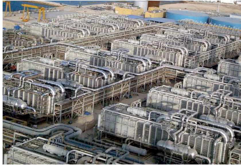
Desalination Plant (S32101, S82122, NSSC2120, S32304, S31803, S32205, S32750, S31254, NSSC270)
